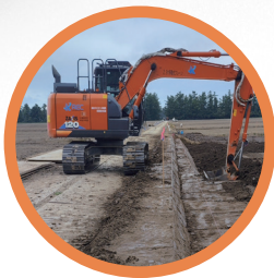
Construction de routes
